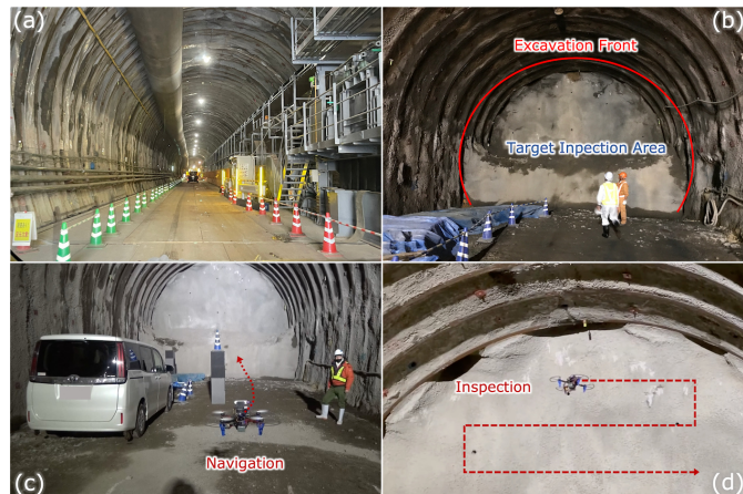
Fig. 1. Illustration of UAV navigating and inspecting the excavation front in the tunnel environment. (a) The tunnel under construction. (b) The target inspection area (the excavation front). (c) The robot navigates toward the inspection target and avoids obstacles. (d) The robot inspects the target area.
