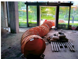
(f) Rigid vent pipe with various cross-section sizes and sharp turns.
