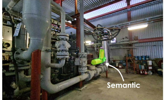
Fig. 1. A flying robot conducting an inspection in an industrial environment.
