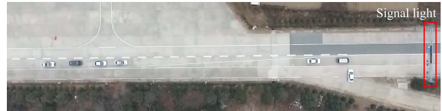
Fig. 5. Top view of the selected road in the test field.
