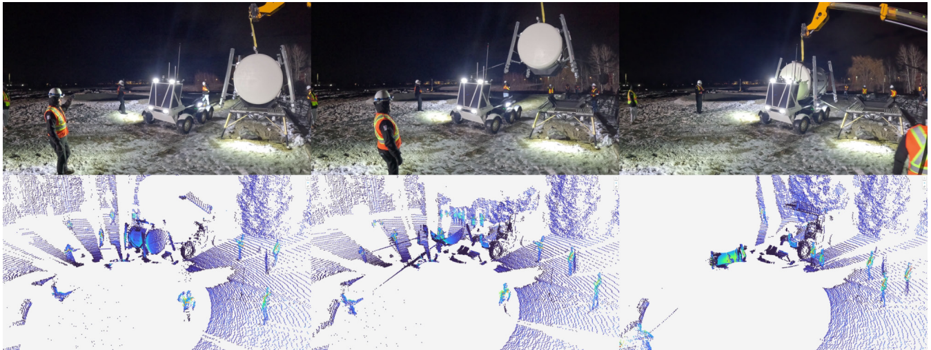
FIGURE 10. Cargo is lifted using the telehandler and loaded onto LELR. The top row is a static camera, and the lower row is the synchronized view from the rover's OS-1 lidar. The high winds required the use of extra personnel with tow lines.
