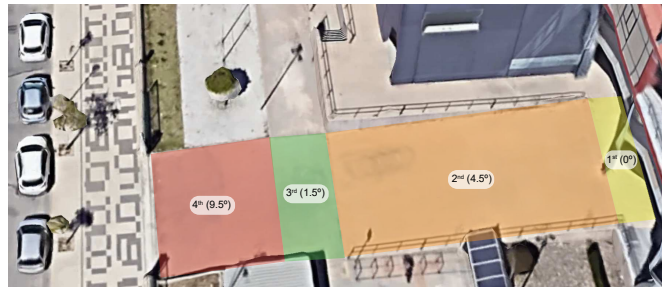
Fig. 5. Photograph of the concrete surface (Google Maps ©2024). Four sloped zones are highlighted and their mean inclination indicated.
