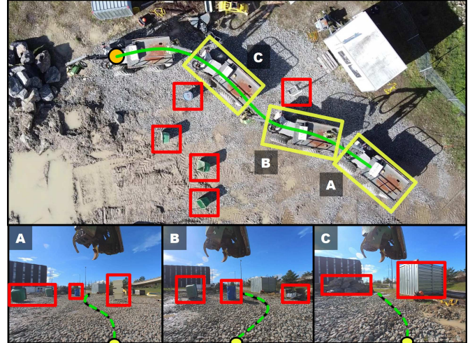
Fig. 1: Experiment of a center-articulated vehicle navigating through a construction site. A, B, and C represent three intermediate moments. The goal is set in the orange dot. The green curve shows the vehicle’s path avoiding obstacles marked by red boxes. The bottom images illustrate how obstacles influence the planning choices.
