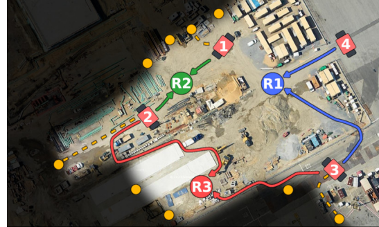
Fig. 1: Robots meeting at rendezvous locations spread over a construction site. The R1, R2, and R3 are hypothetical rendezvous locations. Colored arrows indicate the rendezvous locations. Orange circles are places to explore and dashed lines represent the paths followed by robots.
