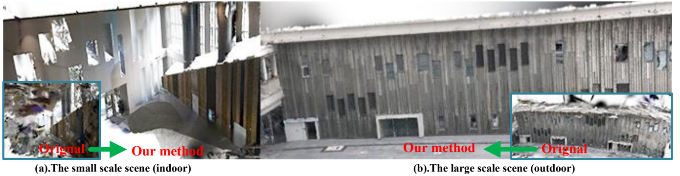
Fig. 2. The figure shows the aerial perspective of the indoor and outdoor scenes of HKUST GZ Tower C1. In contrast to the vision build-up structure by 3D-GS [1], our approach yields a more refined structure with few artifacts.
