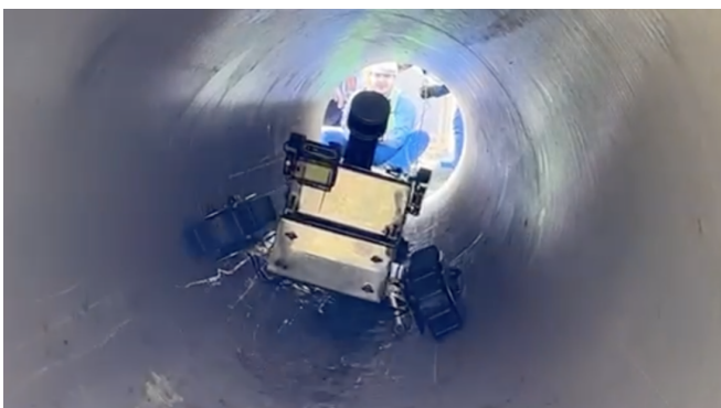
Fig. 5. Validation test in a controlled environment, consisting of a 12 meter fiberglass pipe segment with a 1.5 meter diameter, free of sediment.
