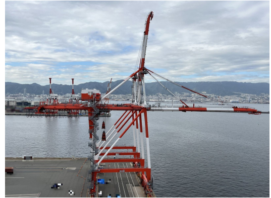
Fig. 1: Appearance of the container crane
